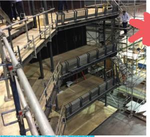
Each of the nine, 35,000-pound "seating towers" are being assembled, level by level, inside The Yard. Together, they create a radically new, adaptable performance arena.
